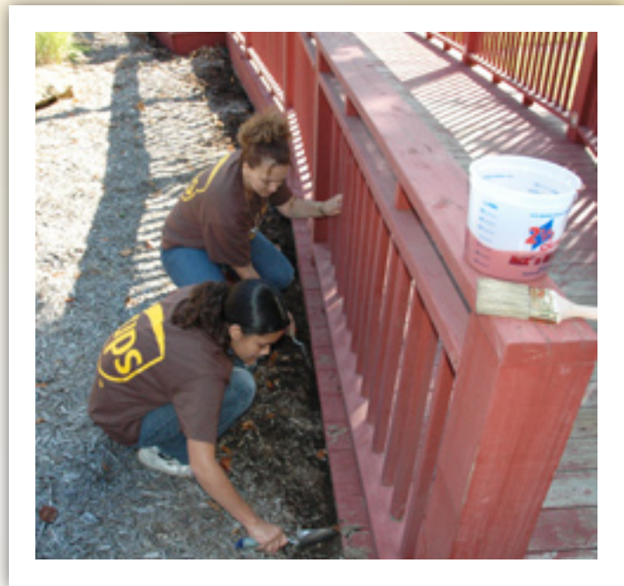
Volunteers from UPS work together to repaint a campus bridge.
